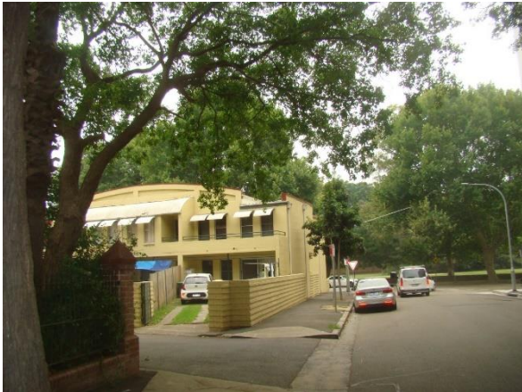
Figure 24. Rear of 2A-2D Wentworth Park Road showing slight elevation, view looking north.
