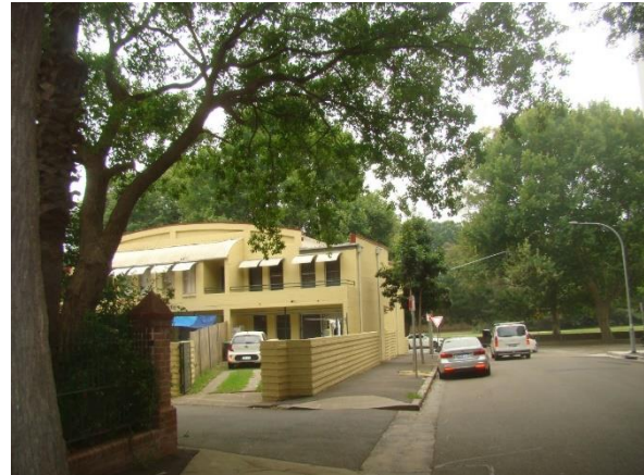
Figure 21. 2A-2D Wentworth Park Road, looking northwest.
