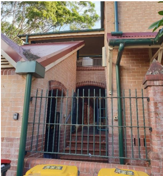
Figure 26. Stairwell at the north access to central courtyard of 17-31 Cowper Street, view looking south.
