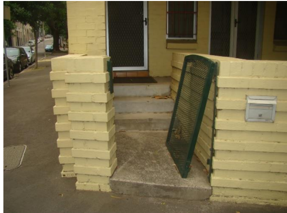
Figure 25. Stairwell at the front of 2A-2D Wentworth Park Road, view looking south.
