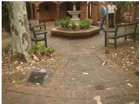
Figure 29. Drainage inlets within the central courtyard of 17-31 Cowper Street.
